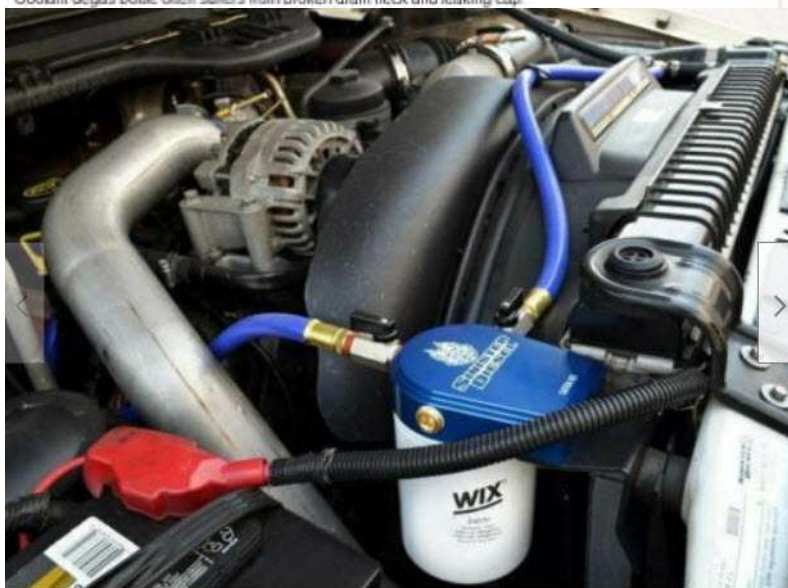
By-pass coolant filter cleans a portion of the coolant continuously
